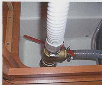
Location of kitchen thru-hull with valve
