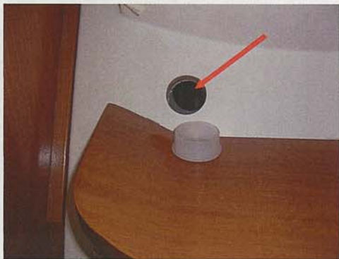
Extinguisher access hole
